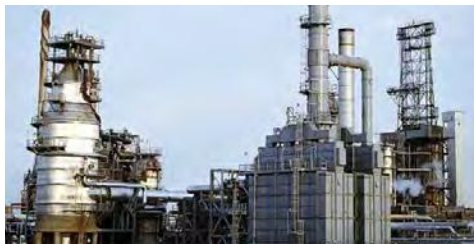
◀ Industrial plants and gas turbine applications
