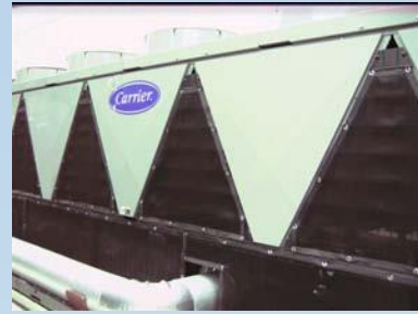
Custom-shaped triangle filters ensure optimum efficiency and simplify maintenance on this Carrier micro-channel coil laboratory cooling equipment in Plano, Texas.
